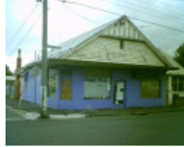
38 Elizabeth Street, Geelong West - Shop
