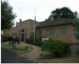
Former Shire of Grenville Offices & War Memorial
