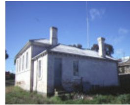
former avoca court house ballarat avoca road avoca rear view aug1984
