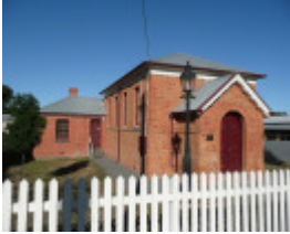
FORMER AVOCA COURT HOUSE SOHE 2008
