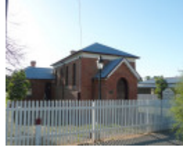
FORMER AVOCA COURT HOUSE SOHE 2008
