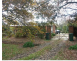
Former Post Office
