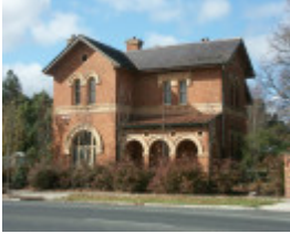
Former Post Office
