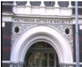
victorian artists society albert street east melbourne detail of front entrance aug1993
