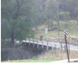
Bridge over Sutherlands Creek
