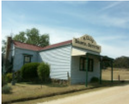
Former Post Office & Shop
