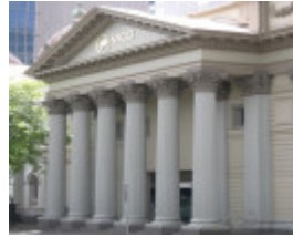
FORMER BAPTIST CHURCH HOUSE SOHE 2008
