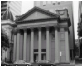
former baptist church house front elevation
