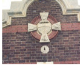
2-4 Selwyn St Elsternwick, September 1994
