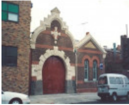
2-4 Selwyn St Elsternwick, September 1994
