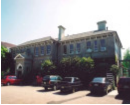
3 Hood Crescent Caulfield North, September 2000
