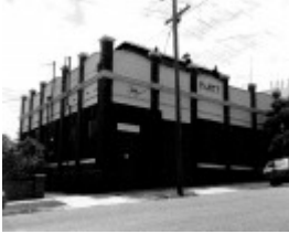
6-8 Rusden Street Elsternwick, August 1994
