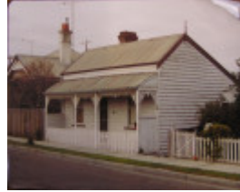
Former dwelling at 199 Autumn Street. Source: GRS1160, Geelong Heritage Centre, c.1981-85.
