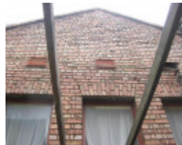
Upper west facade of school Aug2014
