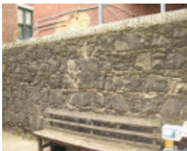
Basalt wall of coursed rubble, west boundary
