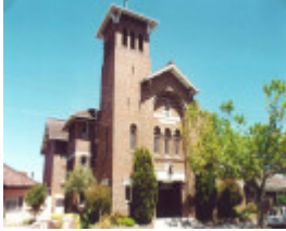
12 Ripon Grove Elsternwick, August 2000
