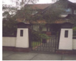
18 Stanley Street Elsternwick, August 2000
