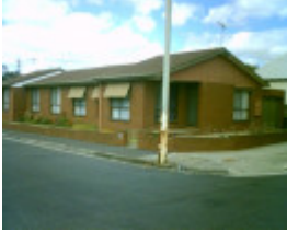
1 Crofton Street, Geelong West - Units
