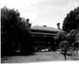
31 Nepean Highway Elsternwick, August 1994
