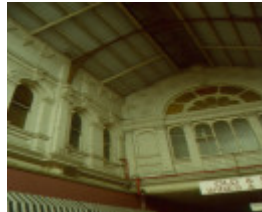
H01960 prahran arcade interior detail 2001
