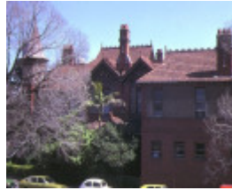
st hildas house clarendon street east melbourne front view roof line
