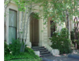
philadephia robertson house clarendon street east melbourne entrance oct1999
