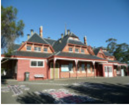
PRIMARY SCHOOL NO. 4 SOHE 2008
