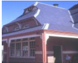
h01622 primary school no 4 barnett st avoca classroom
