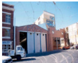
Former Hawthorn Tramway Depot During Redevelopment
