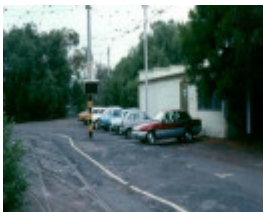
Former Hawthorn Tramway Depot Fan and Tower Wagon Shed
