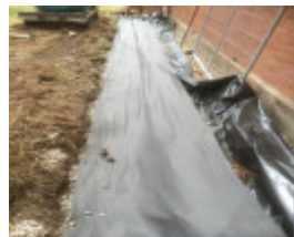
During Photograph - Reference F3878 2015
