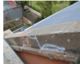
Before Photograph - Reference F3878 2014
