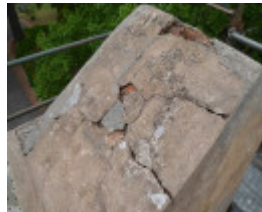
Before Photograph - Reference F3878 2014
