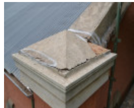
Before Photograph - Reference F3878 2014
