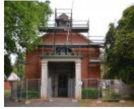
During Photograph - Reference F3878 2015
