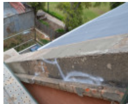
Before Photograph - Reference F3878 2014
