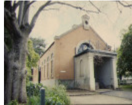
1 former market hall & royal oaks high street maldon side view aug1997
