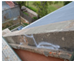
Before Photograph - Reference F3878 2014
