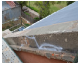
Before Photograph - Reference F3878 2014
