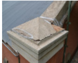
Before Photograph - Reference F3878 2014
