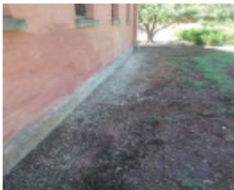
Before Photograph - Reference F3878 2014
