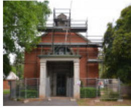
During Photograph - Reference F3878 2015
