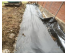
During Photograph - Reference F3878 2015
