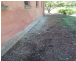
Before Photograph - Reference F3878 2014
