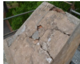
Before Photograph - Reference F3878 2014
