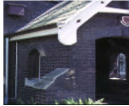
st peters church and vicarage exterior entrance
