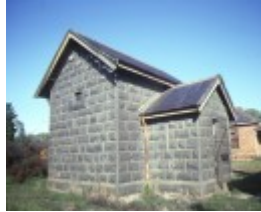
1 lock up davey street avoca side view aug1984
