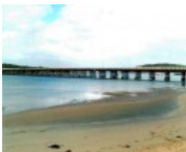
1 barwon river bridge ntv
