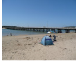
BRIDGE, BARWON HEADS SOHE 2008
