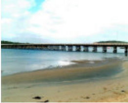
1 barwon river bridge ntv
