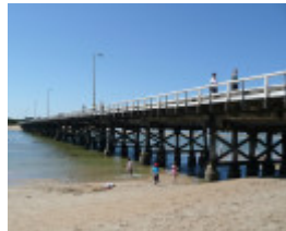
BRIDGE, BARWON HEADS SOHE 2008
