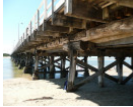
BRIDGE, BARWON HEADS SOHE 2008
