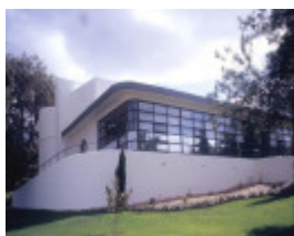
former hamilton tuberculosis chalet tyers street hamilton view from carpark entrance she project 2003
