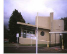
1 former hamilton tuberculosis chalet tyers-street hamilton side elevation aug1994
