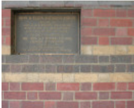
RETAINING WALL SOHE 2008
