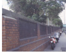
1 flinders street extension retaining wall street view mar1999
