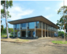
FORMER BP REFINERY ADMINISTRATION BUILDING SOHE 2008
