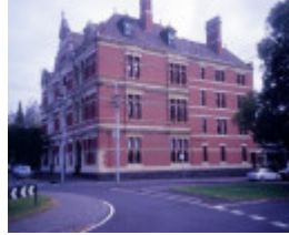
h00602 queen bess row hotham st east melbourne cnr view
