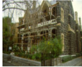
157 hotham street verandah restoration
