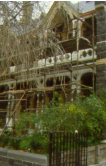
157 hotham street verandah restoration
