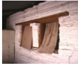
1 blue cottage/pise cottages zumsteins blue cottage window detail
