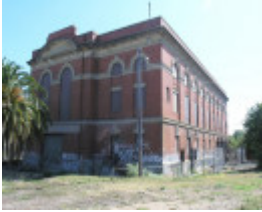
RAILWAY SUB-STATION SOHE 2008
