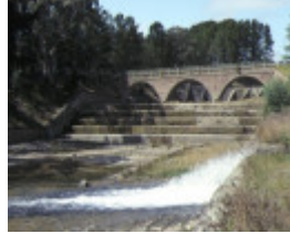
1 coliban water system bendigo spillway mar1993
