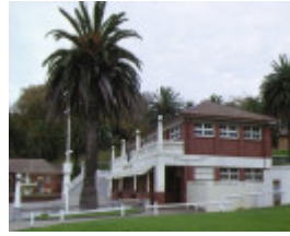
1 eastern beach bathing complex & reserve geelong cafe side view
