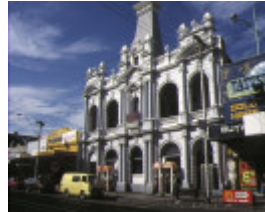
1 former collingwood post office smith street collingwood front elevation mar1993
