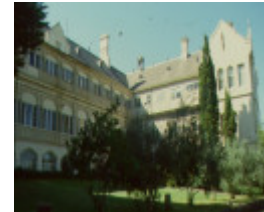
1 little sisters of the poor northcote front 2001
