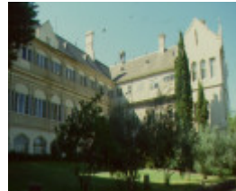
1 little sisters of the poor northcote front 2001
