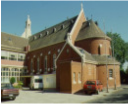
Little Sisters of the Poor Northcote Chapel 2001
