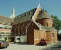
Little Sisters of the Poor Northcote Chapel 2001
