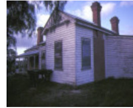
former police residence davey street avoca rear view
