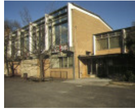
1 beaurepair centre university of melbourne parkville exterior view jul1993
