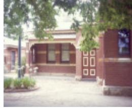
h01070 former benalla court house arundel street benalla old witness room she project 2004
