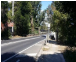
Chandler Highway Bridge looking to the south (City of Boroondara) from the northern side of the bridge (City of Yarra).jpg
