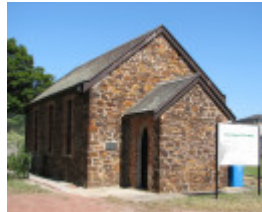
FORMER ST JOHN'S THE LESS ANGLICAN CHURCH AND SCHOOLROOM SOHE 2008
