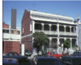
1 terrace 20 & 22 morrison place east melbourne front view nov1990
