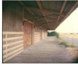
h02072 port fairy goods shed platform
