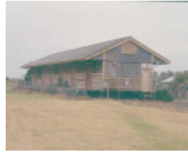
h02072 port fairy goods shed
