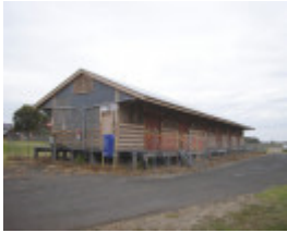
RAILWAY GOODS SHED SOHE 2008
