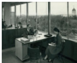
ICI House - An Interior Office 1958 Photo by Wolfgang Sievers.JPG
