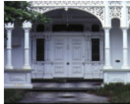
Eastcourt Powlett Street East Melbourne Detail Entrance
