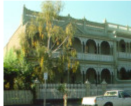
Eastcourt Street Facade May 2001
