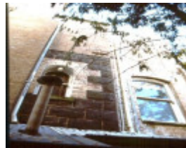
138 powlett street east melbourne h89 south elevation
