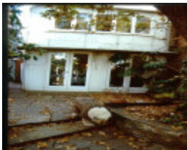
138 powlett street east melbourne h89 rear may2000
