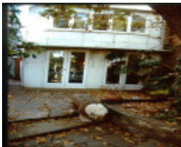
138 powlett street east melbourne h89 rear may2000
