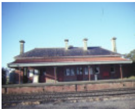
avoca railway station york avenue avoca front view aug1984
