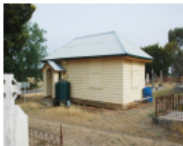
MALDON ROAD TOLL BAR HOUSE SOHE 2008
