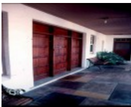
H01998 bruce manor frankston rear verandah
