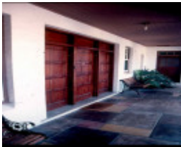
H01998 bruce manor frankston rear verandah
